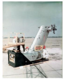
The crew 1 bolt removal man installed the main transmission sling, while crew 3 was preparing the main transmission for removal. The engine drive shafts were removed, tail rotor drive shaft unhooked, and main
